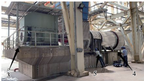
图 6 4 台一次风机混凝土基础测点布置 Fig.6 Layout of measuring points of concrete foundation of four primary air fans
