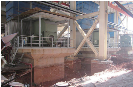
图 3 4 台一次风机混凝土基础外侧区域开挖实物图 Fig.3 Physical drawing of excavation outside concrete foundation of four primary air fans
